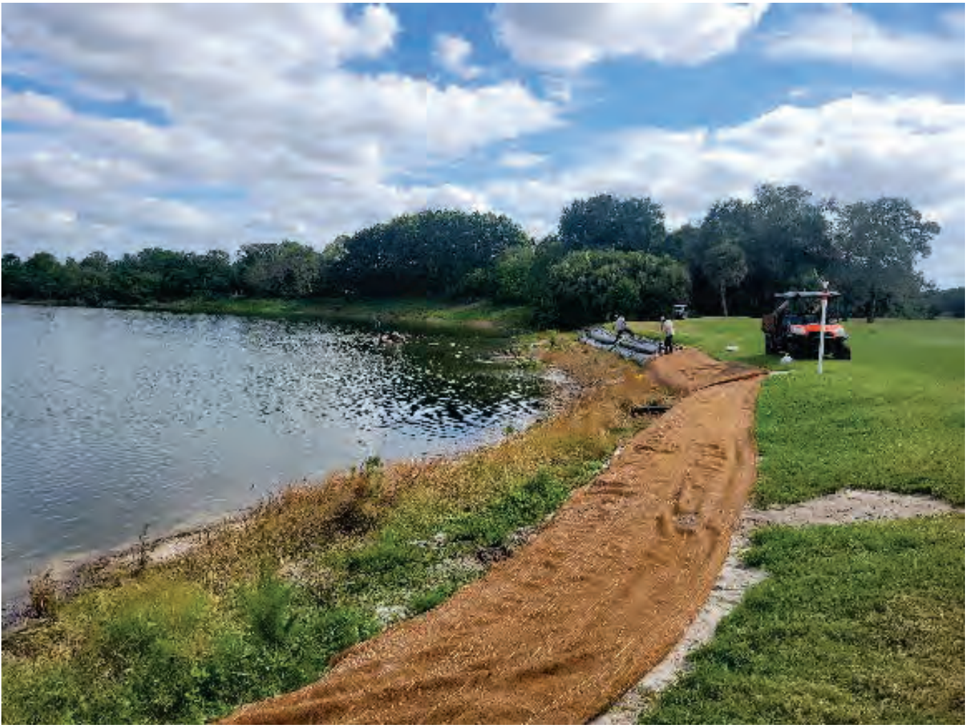
Coconut Coir TRM (If used) prior to sod
