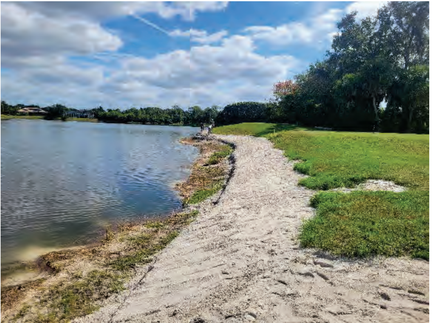
Final hand graded shoreline prior to Coconut Coir TRM and/or Sod
